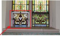
These two ventilators have been placed in the wrong location years ago when the ventilators were updated. We will be swapping these two ventilators back when the restoration is being completed.
