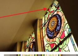
If you look closely at a few of your windows, you will see that some have begun to bow. This is due to the fact that the lead, solder, and cement are in a deteriorated state.
