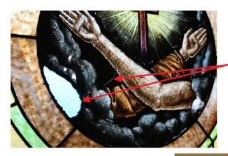
Here is a symbol that has been broken for some time. We will replace this with a new symbol using our progressive painting system where we can digitally re-master the piece for the most accurate duplication.
