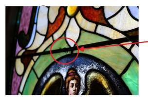
Numerous areas around the church have broken tie wires. Once these tie wires break away from the stained glass, the windows begin to bow at an accelerated pace. This eventually leads to glass breakage. We recommend restoring your windows before this becomes a more expensive repair in the future.
